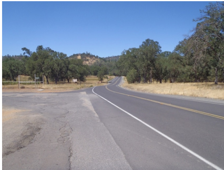
Figure 18. Key View 2—Existing Condition Facing Westbound
