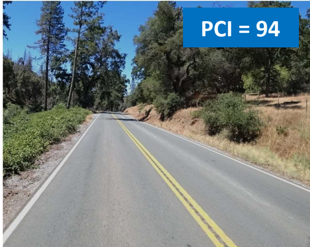
Mountain Ranch Road between Boo St and Brothers Rd
