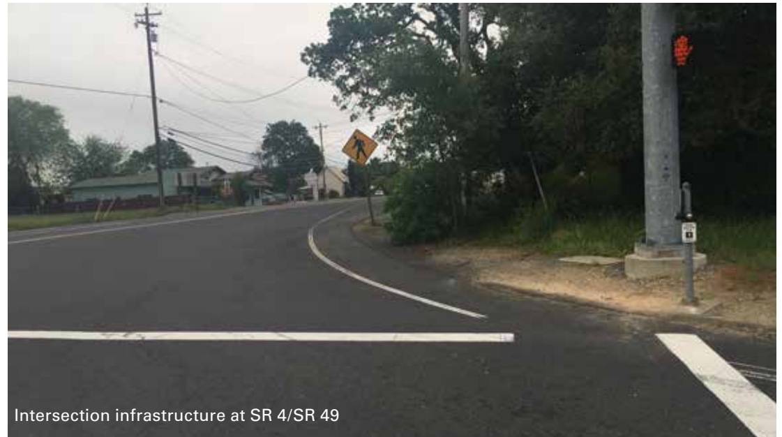
Intersection infrastructure at SR 4/SR 49
