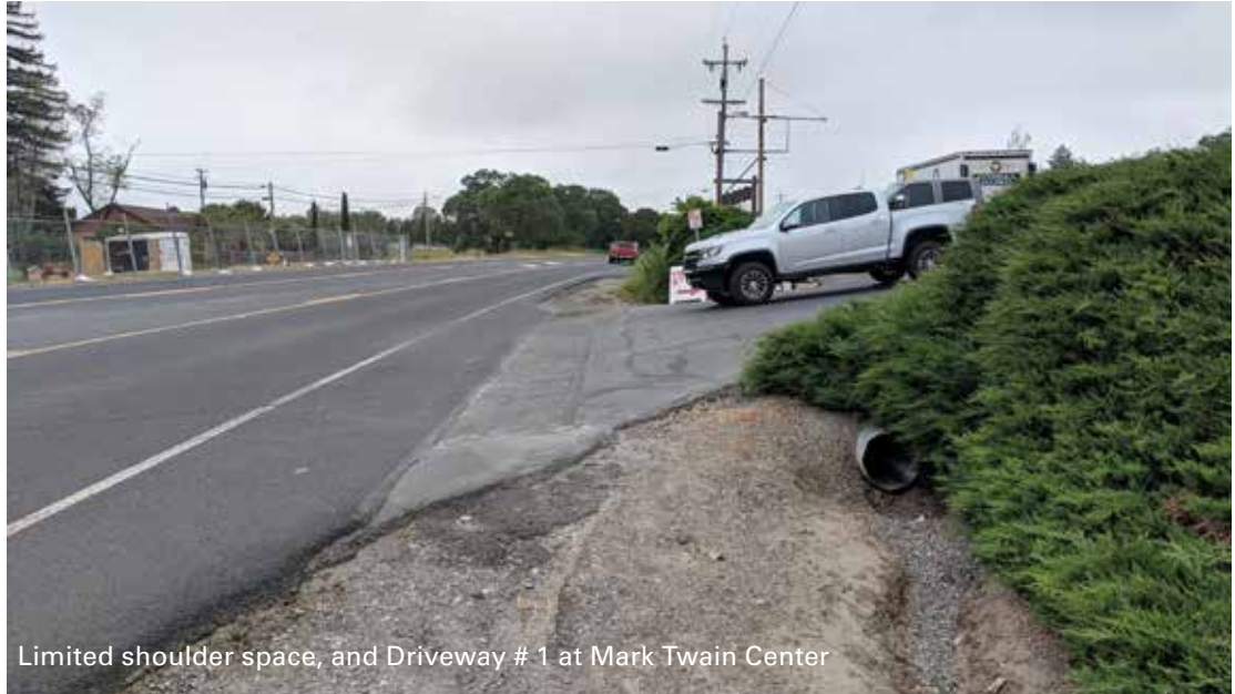
Intersection infrastructure at SR 4/SR 49
