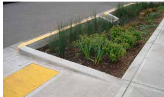
Curb-cuts with brightly colored rumble strips
