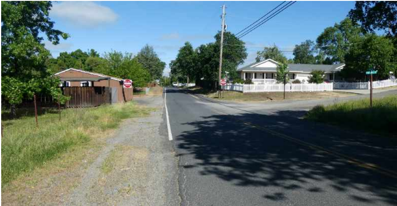
Lewis Avenue facing west near Foothill Court. Lewis Avenue is characterized by narrow/non-existent shoulders.
