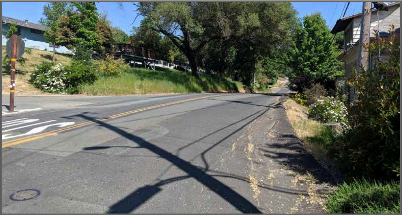
Intersection of Pope Street and California Street facing east with no shoulder.
