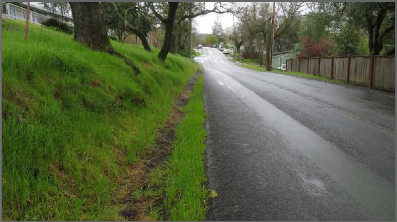
Desire line along Pope Street where there is no shoulder nor sidewalk.
