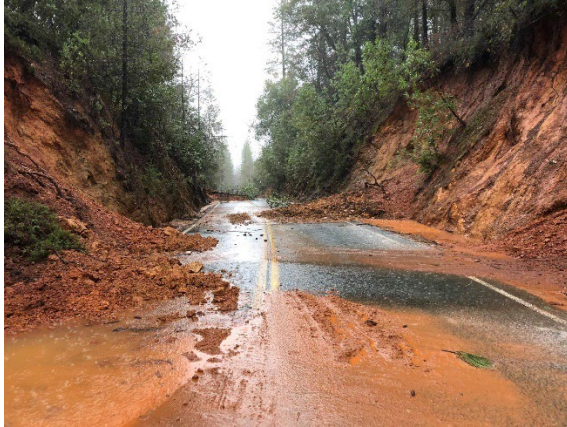
Figure 5. Image from Highway 26 Road Closure near Mokelumne Hill 6
