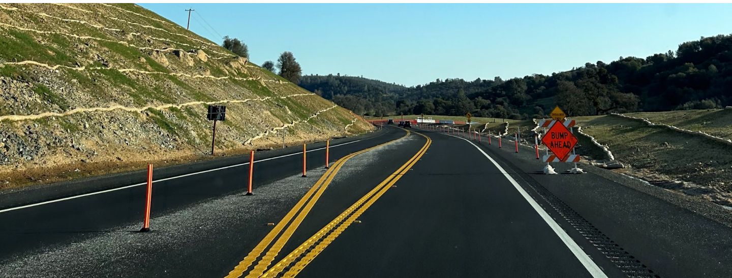
Figure 6.2 Photo of State Route 4 Wagon Trail Project
