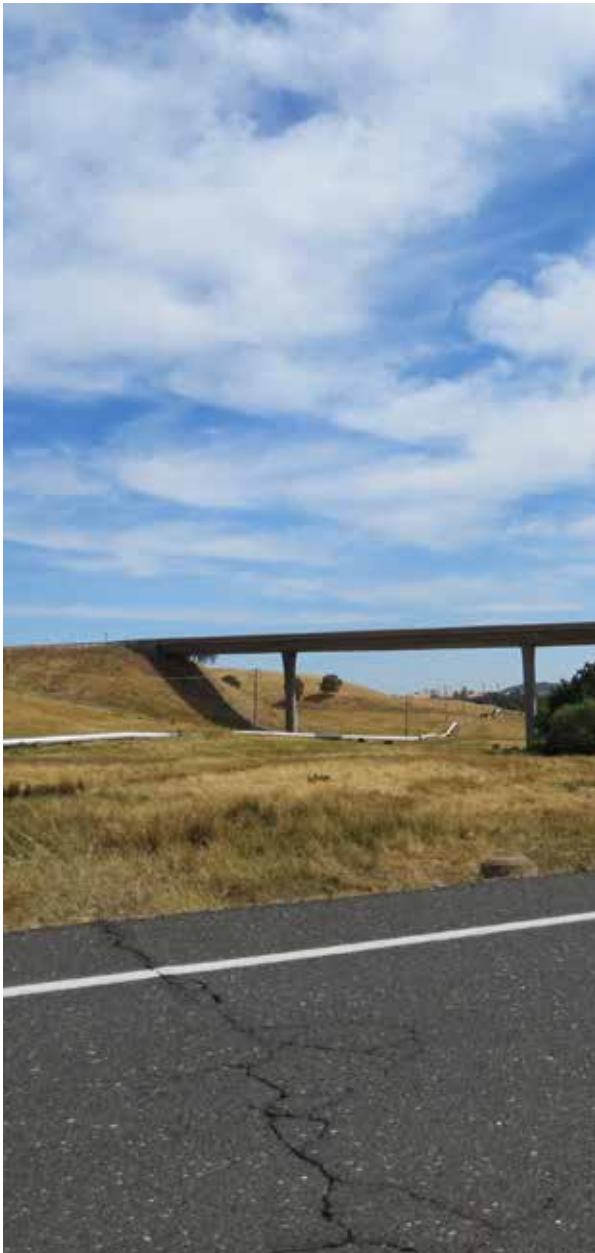
SR4 Bridge from Murphys Grade Road
