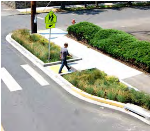
Example of pedestrian intersection with bump out for traffic calming, signage, ADA ramp and high visibility pavement markings.
