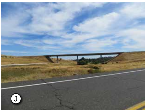
SR 4 bridge towards Murphy's from Murphys Grade Road
