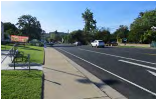
Existing Sidewalk along SR 49 in Angels Camp
