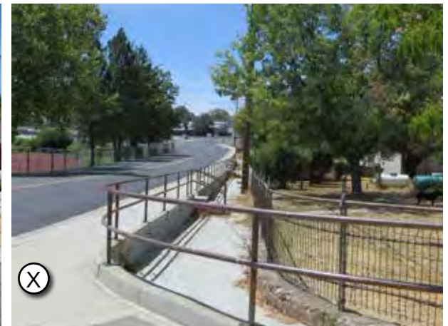
Gardner Lane and Murphys Grade toward High School
