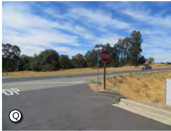
Foundry Lane/SR 4 intersection
