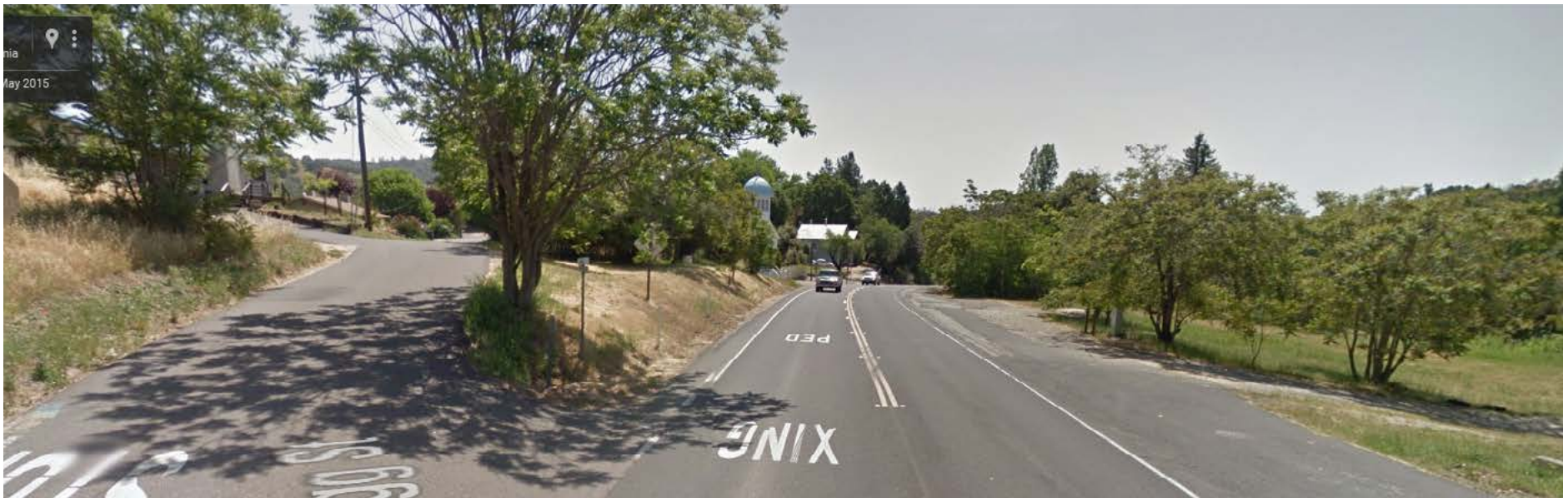
Existing Bragg Street Intersection
