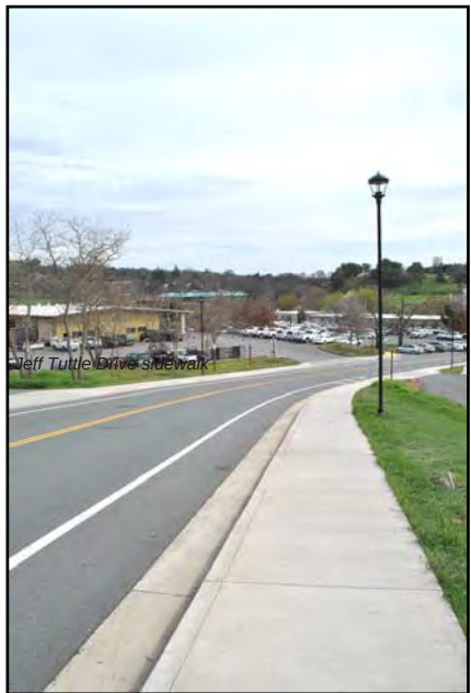
Government Center Drive sidewalk - South Direction
