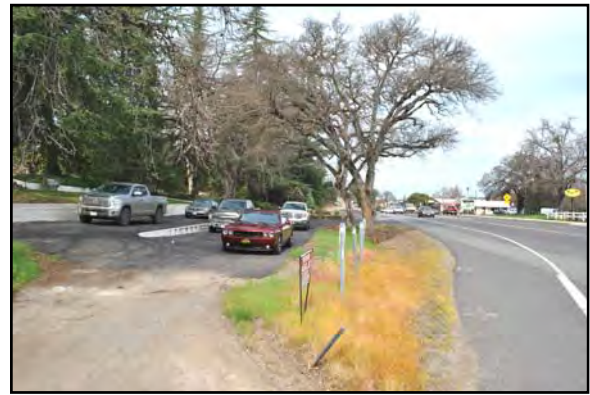
Lack of sidewalk in the southbound direction on SR 49
