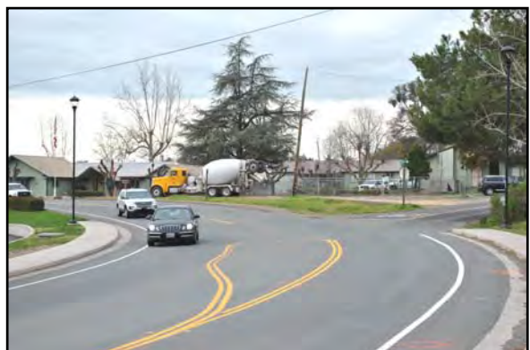
Approaching Mountain Ranch Road/Pope Street intersection from the East
