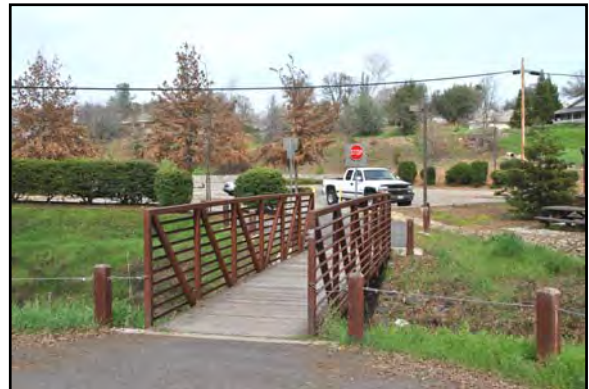
Pedestrian bridge crossing at the Public Library
