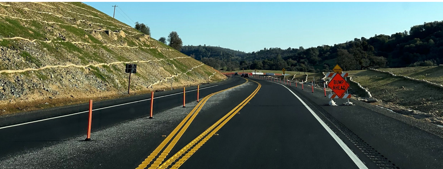
Figure 6.2 Photo of State Route 4 Wagon Trail Project
