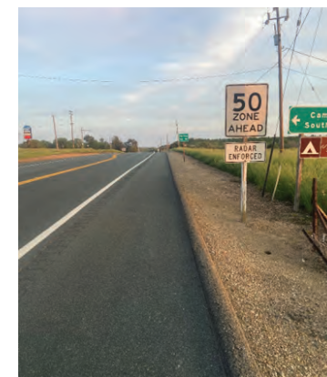
Paved Shoulders with Rumble Strips on SR 12 in Wallace, CA. Source: Fehr & Peers, 2025
