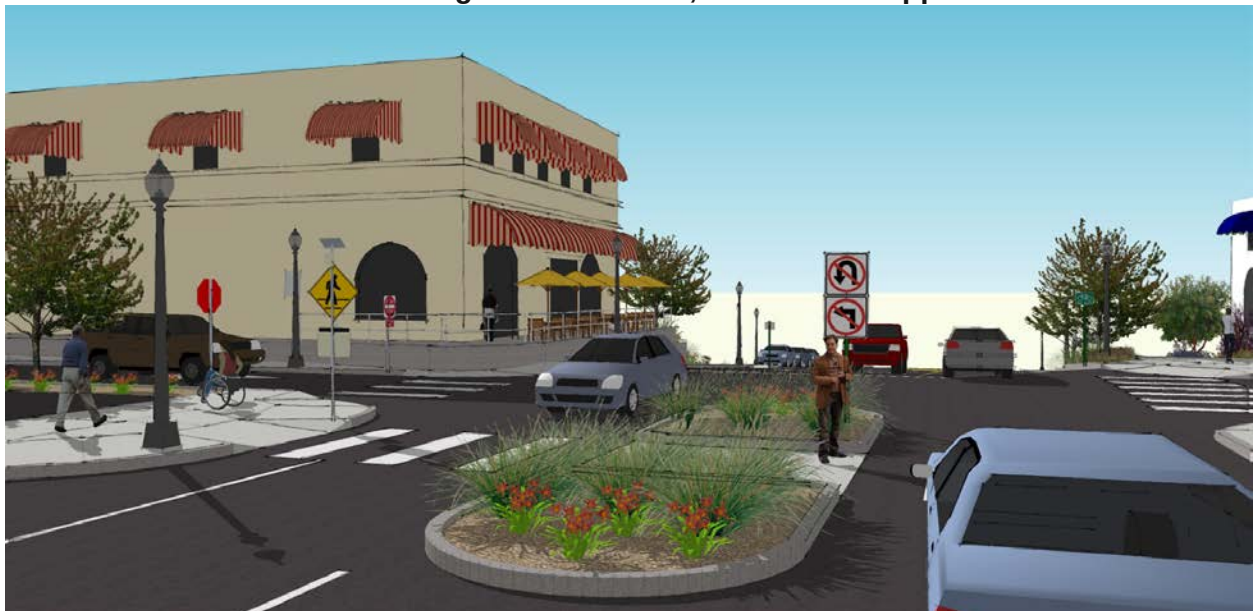
Pedestrian Refuge at Main Street, Northbound Approach
