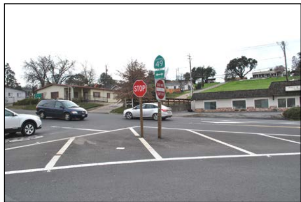
SR 49/Mountain Ranch Road intersection
