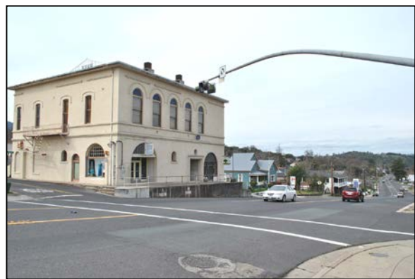
SR 49 /Main Street intersection
