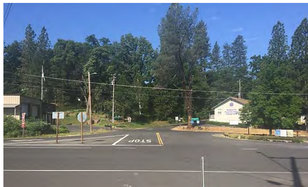
Existing Main Street/Jones Street/SR 4 intersection
