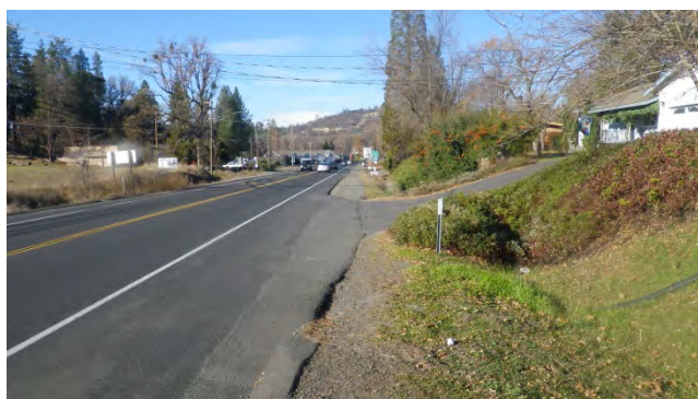
Existing shoulder on central SR 4, looking east
