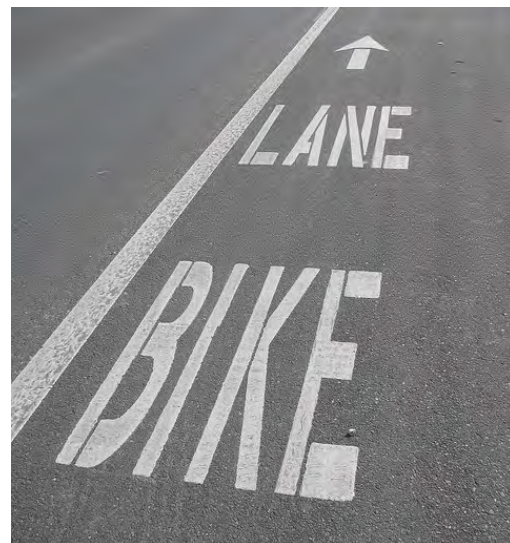
Class II bike lane pavement markings
