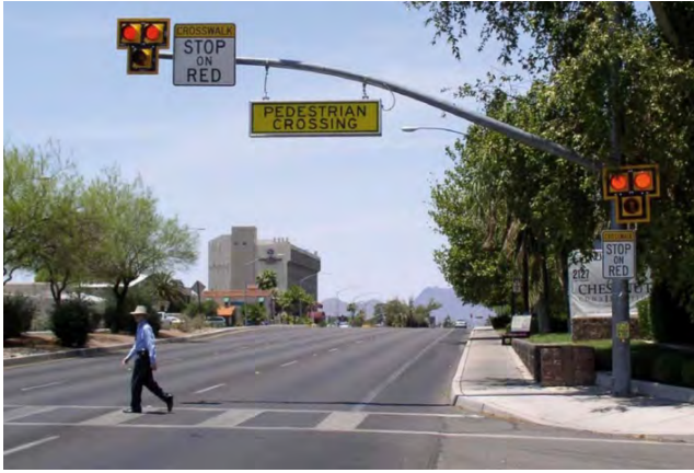
High visibility pedestrian crossing and pedestrian crossing beacon
