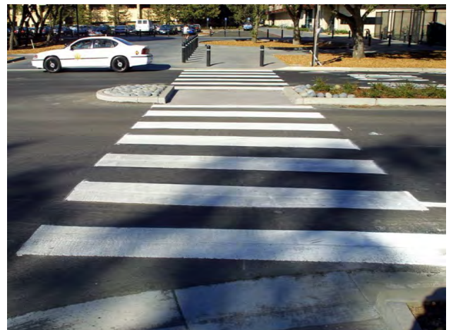
High-visibility crosswalk with pedestrian refuge island
