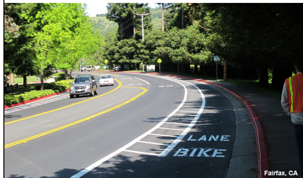
Buffered Bike Lanes and Central Turn Lane
